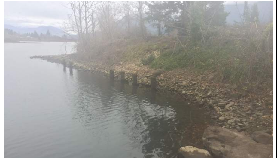
Photo 4. Riprap on the eastern shoreline, facing south.
