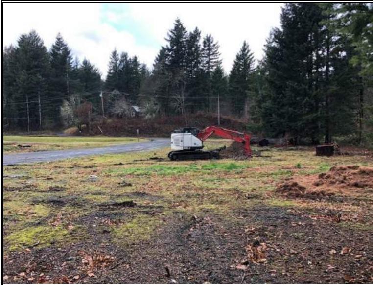
Excavation of test-pit TP-3, looking west
