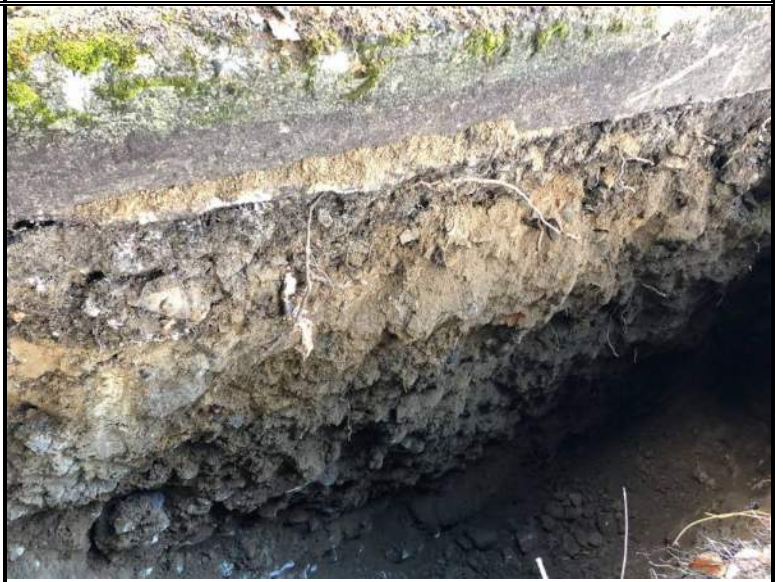
Exposed subsurface soil profile within test-pit TP-6
