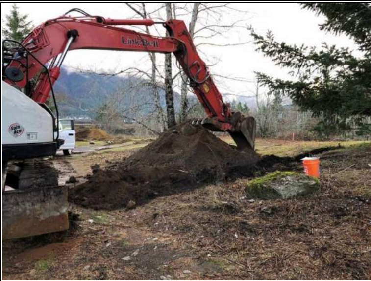
Exposed subsurface soil profile within test-pit TP-11
