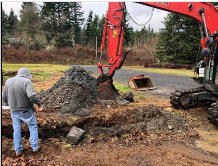
Excavation of test-pit TP-1, looking west
